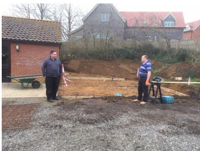
Socially distanced work in progress.....
